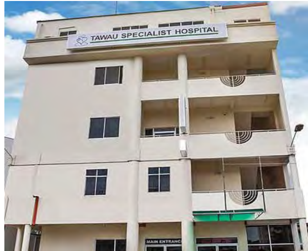
Figure 14.8. Tawau Specialist Hospital
