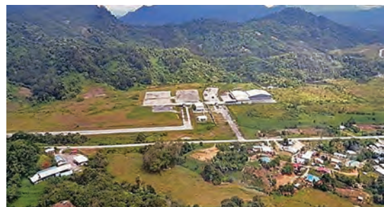
Figure 8.5. Aerial View of Tebedu Inland Port
